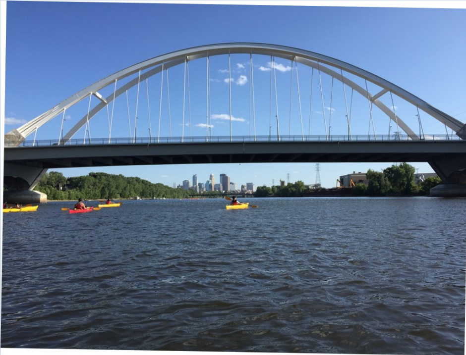
Minneapolis Lowry Bridge
