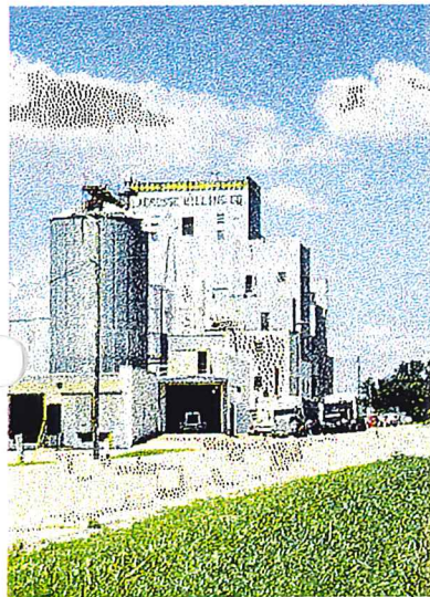
Grain elevators help process, store, and load grain
