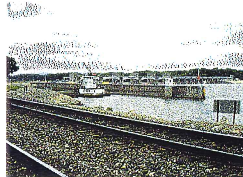
A tugboat pushes a barge into the lock at Lock and Dam No. 9
