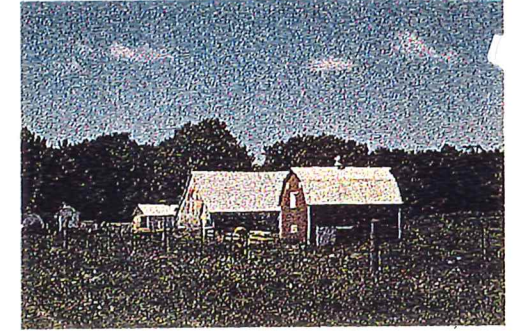
Gambrel roofs provide more hay storage space than gable roofs
