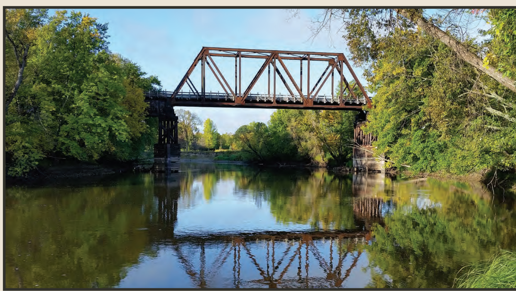
Soo Line Bridge in Palisade
