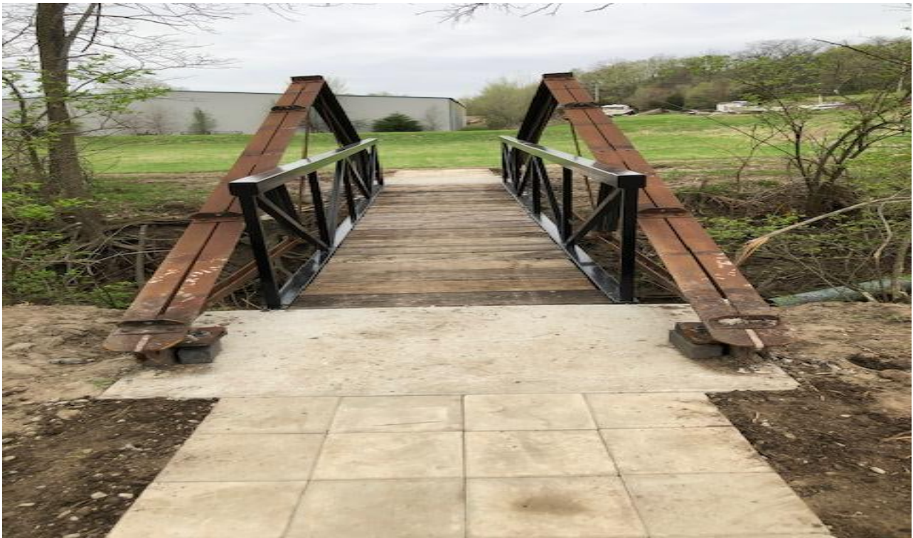
Figure 10. Photograph of new replacement bridge on South Trail, showing trusses salvaged from original Pumphouse roof reused as decorative element in bridge design.
