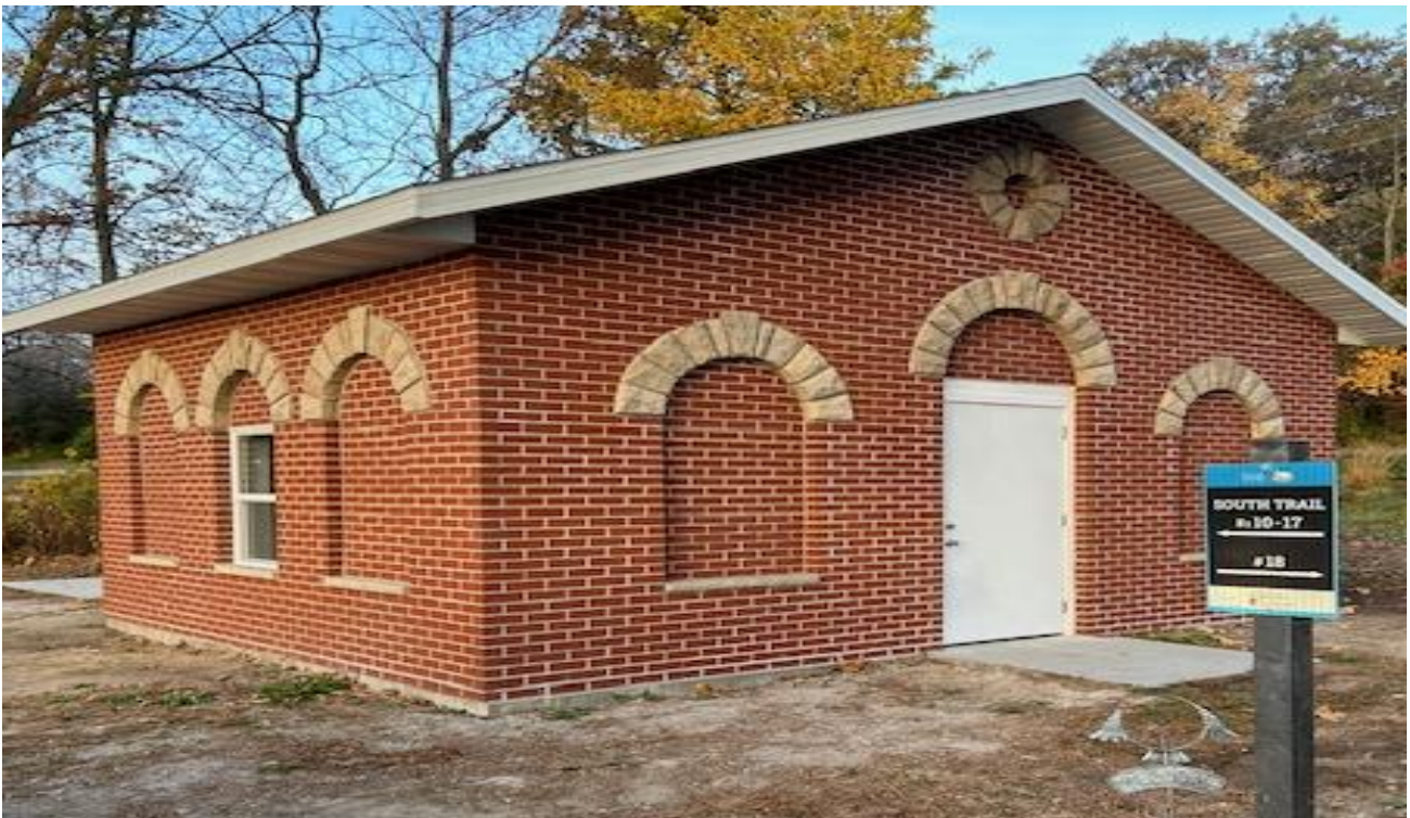
Figure 9b. East view of the Pavilion, note salvaged sandstone blocks used for bullseye, door and window arches.
