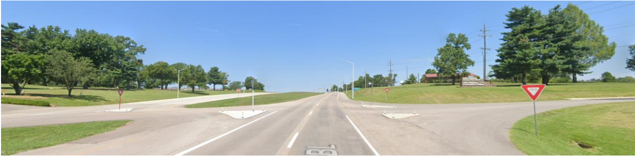
Northbound, I-55 Business Loop/US 61 North/GRR, at signage on roadway absent, site sign to right
